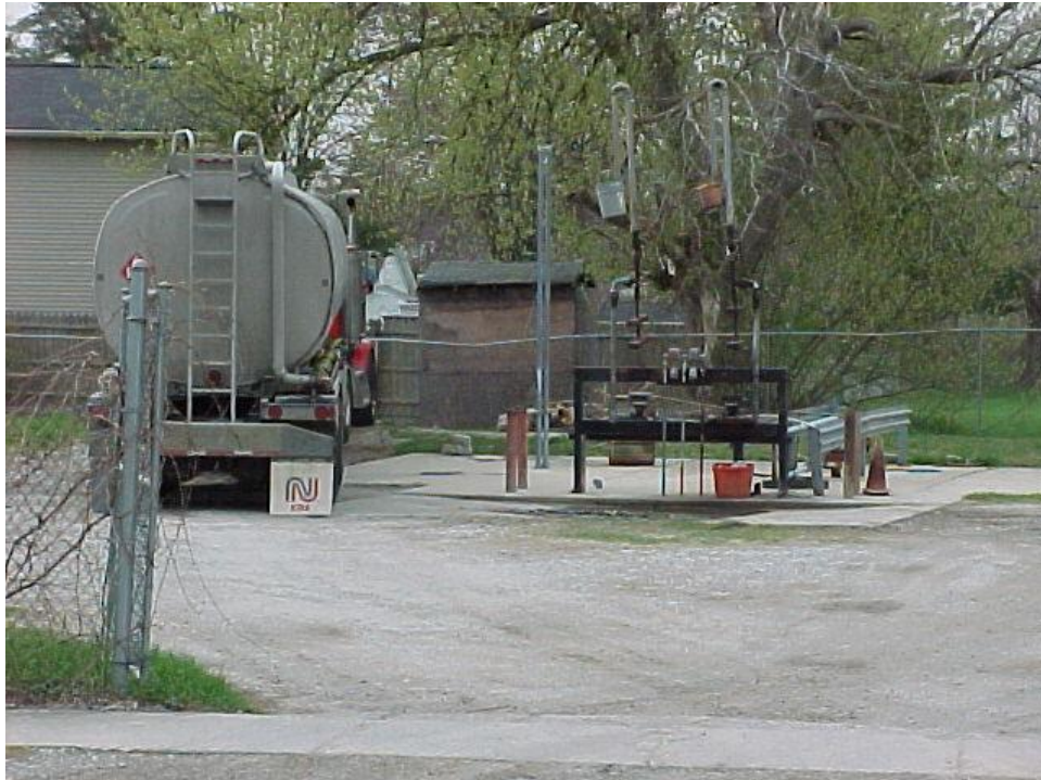
Picture of Ken's Oil Bulk Plant.
